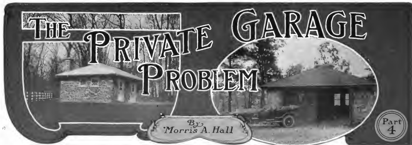
Two Examples of Stone Construction, One, Rubble Stone Laid in Concrete, the Other, Field Stone Laid as Broken Ashlar
